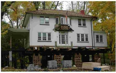
During the past several years, the Delaware River has flooded with increased frequency and caused damage to many homes along its banks, particularly in Yardley, PA. As a result, many homeowners in this area have sought the services of home lifting companies. Structural engineering services are also required for the design of the new bearing walls and frames, which will ultimately be in place to support the home in its final raised position.
